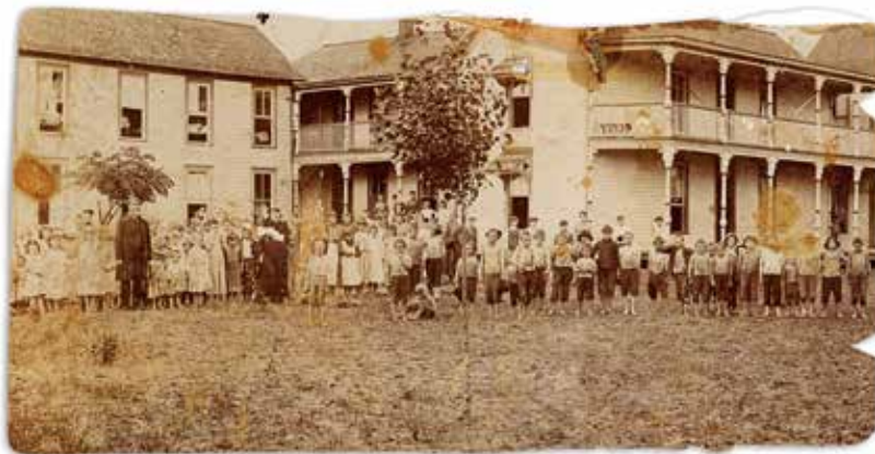
In the only known photograph of the original buildings, children pose with R.C. "Father" Buckner (at left), on the Buckner Orphans Home campus. The building at right burned in 1897.
